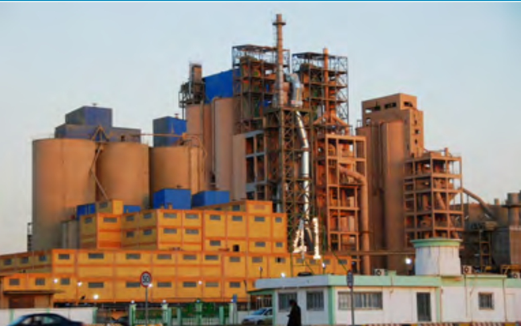
□ Asamer cement factory in Benghazi
