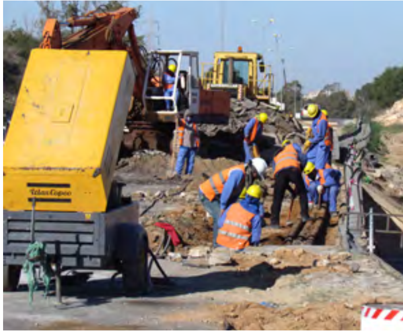
□ Repairing Nageza bridge
